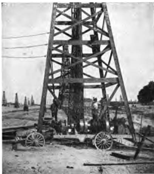
FIG. 66. Portable electric pulling machine (Westinghouse).
