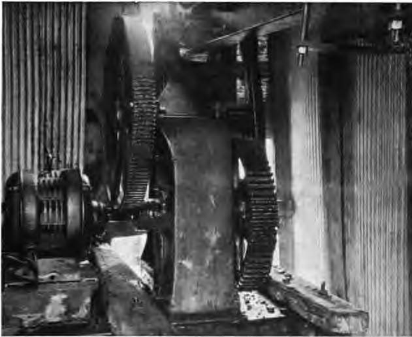
FIG. 61. Westinghouse electric motor connected to pump individual well.
