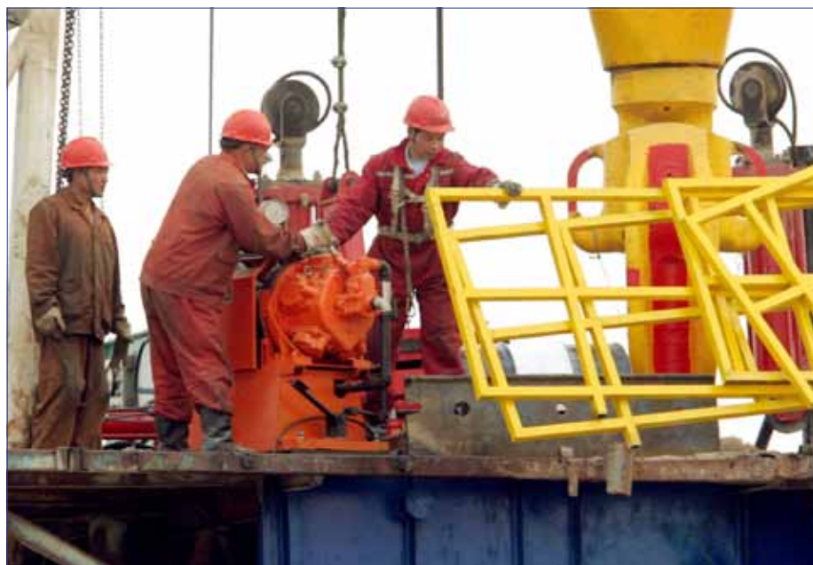
Construction works at a PetroChina oil well in Lunnan, Xinjiang
