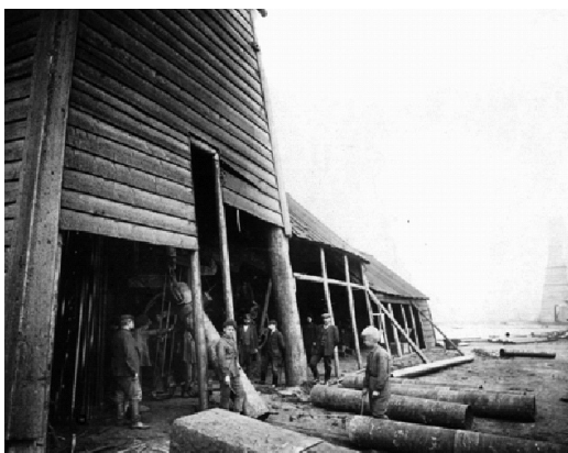
The lifting of pipes for riveting in the well
