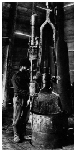
A drilling bit with an expander
