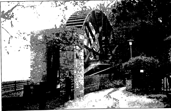
An oblique view of the water wheel together with the jerker line system for pumping brine well.
