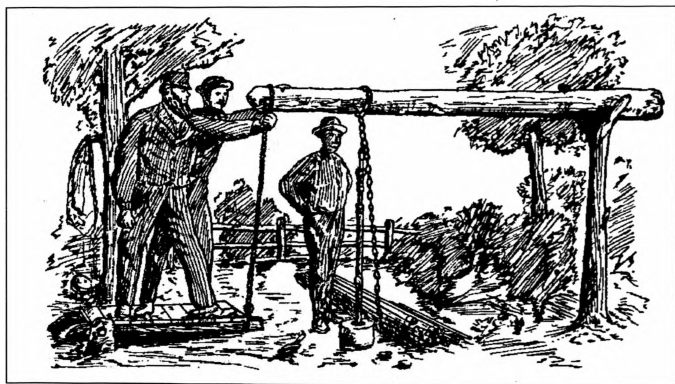
Spring pole detail with a platform for "kicking down" the hole.
