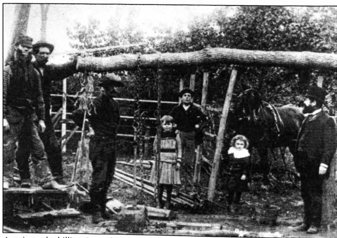
A spring pole drilling rig used in the Petrolia fields.
