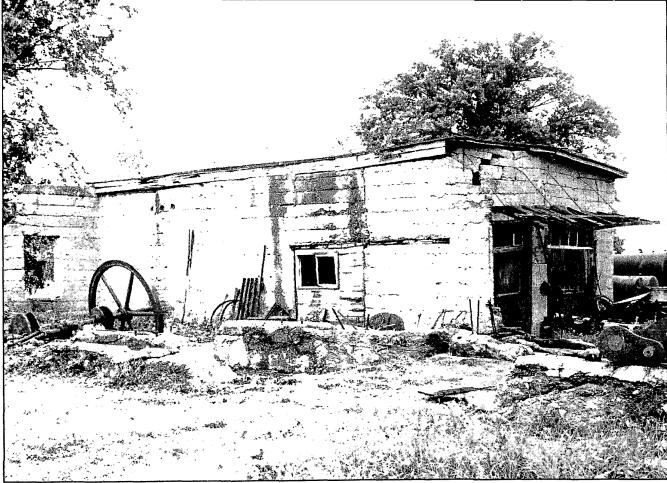
The boiler house for the original steam powered jerker line system with the ruins of the engine shed in the foreground
