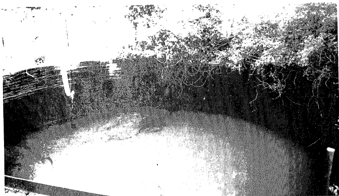
A large underground tank for receiving oil from a number of wells pumped with the jerker line system.
